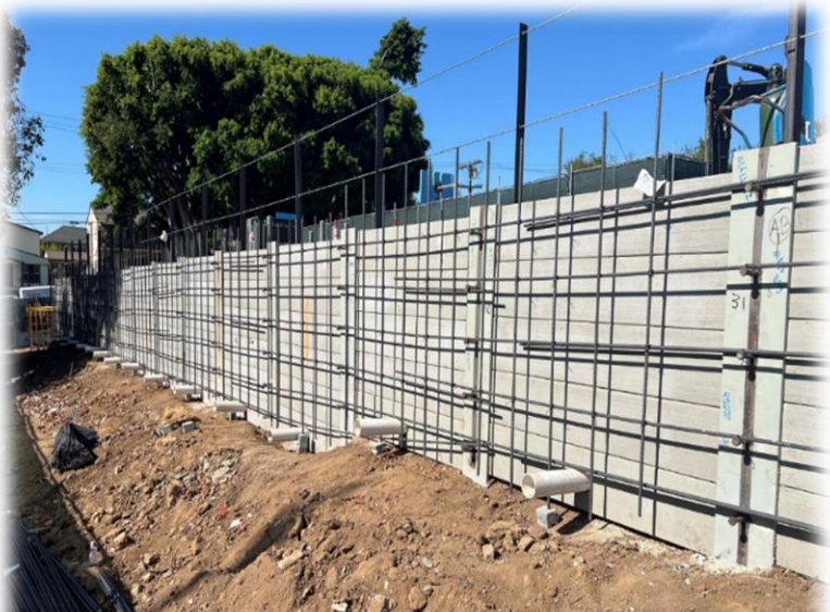
Face of Retaining Wall with Concrete Lagging & Rebar
